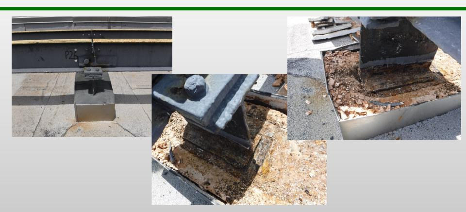
Roof Carriage Track: System in place for many years and had been previously tested. Track had never been welded down in one location.
